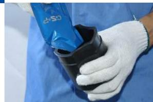
Fill approximately half the grease supplied into the joint
